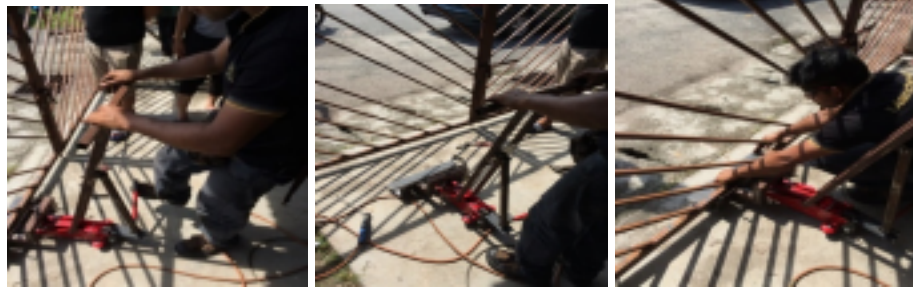
Figure 6: Installation work using tools.
